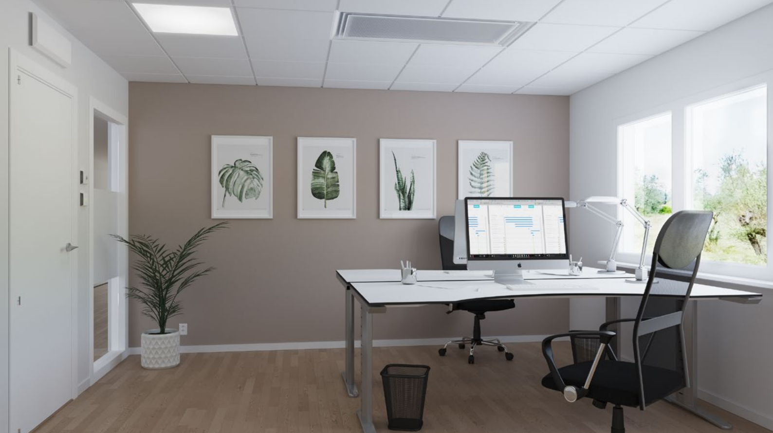
Waterborne office with setpoint selector switch and occupancy sensors for demand-controlled ventilation, cooling and heating.
